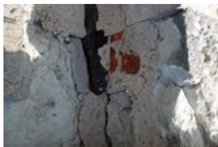
Above: Crumbling stone work on the tower.
